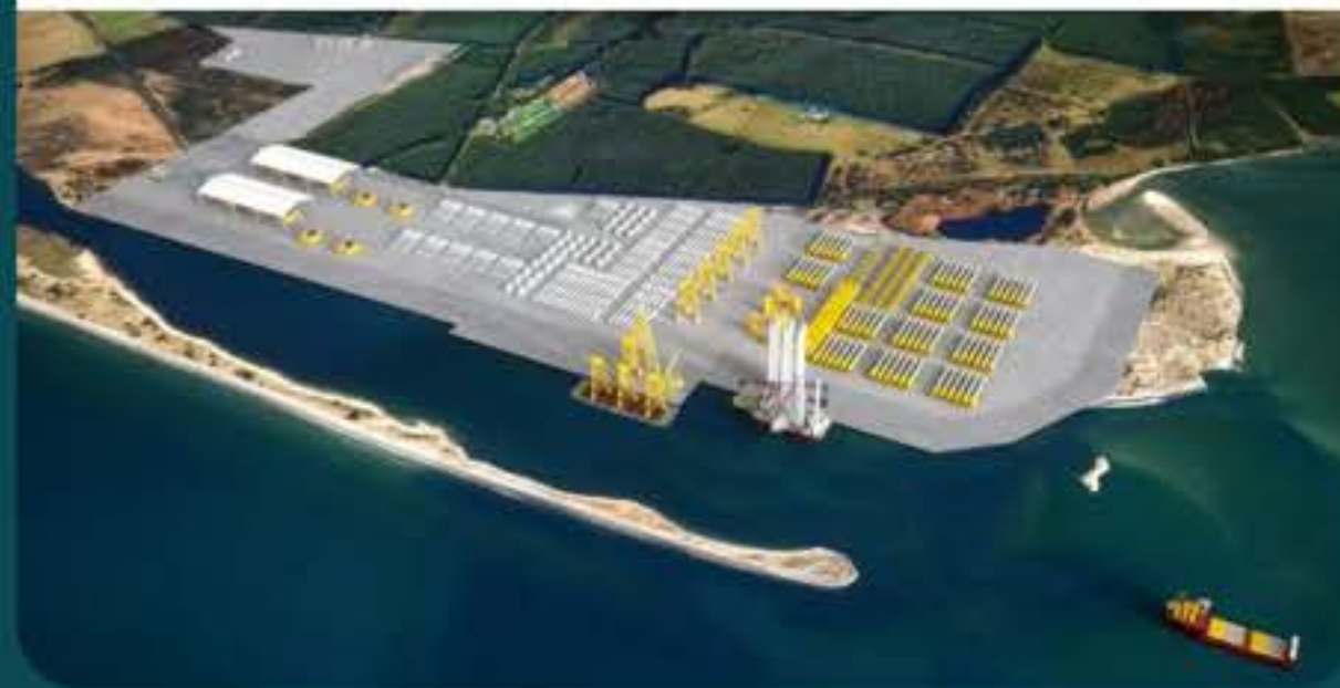
Ardersier Energy Transition Facility
