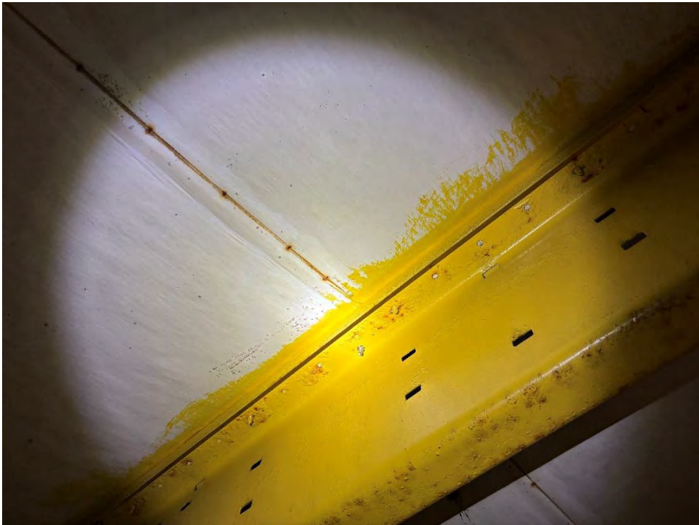
Photo 4 – Typical Roof Purlin in Hockey Rink Showing Minor Corrosion Staining on the Top Flange.
