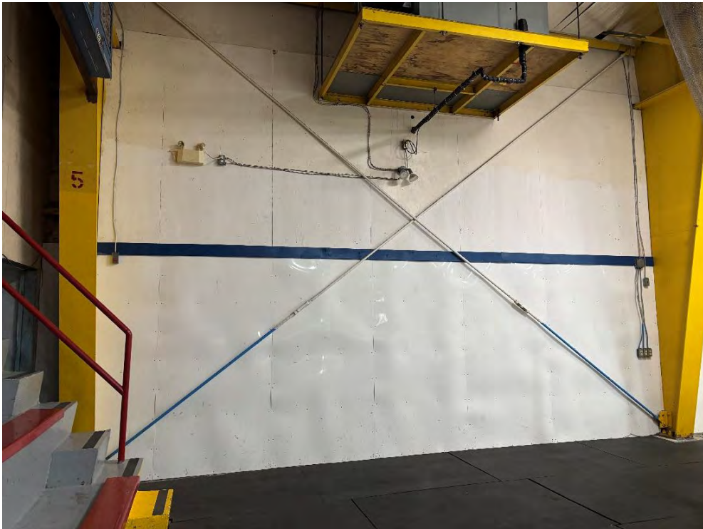
Photo 8 – Rigid Frame Columns and Vertical Rod Bracing Along South Wall.
