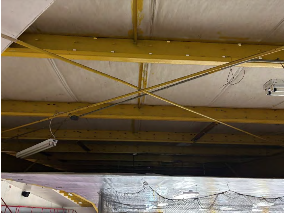
Photo 7 – Typical Lateral Rod Bracing in Roof Structure.
