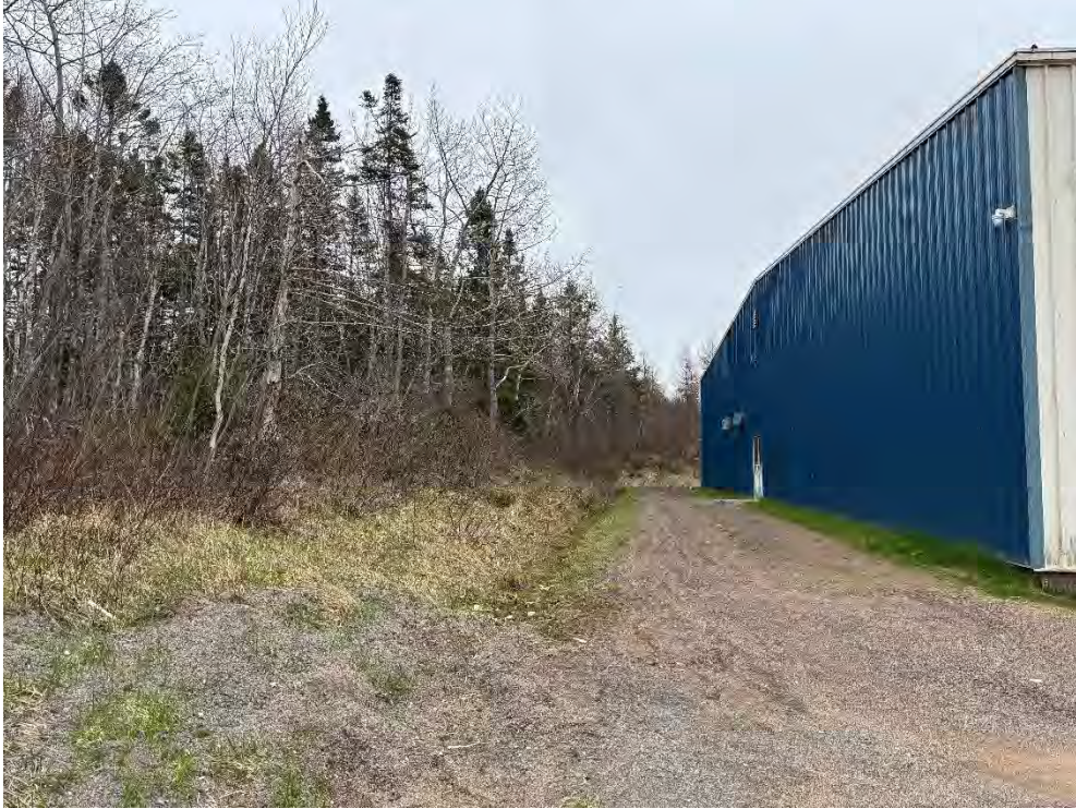
Photo 15 – Exterior View Along East Side of Building.
