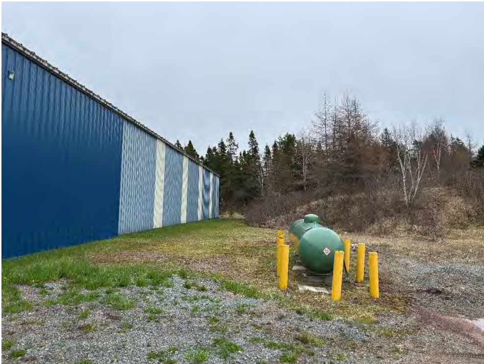
Photo 16 – Exterior View Along South Side of Building.
