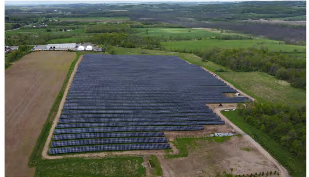
Community Solar Project
