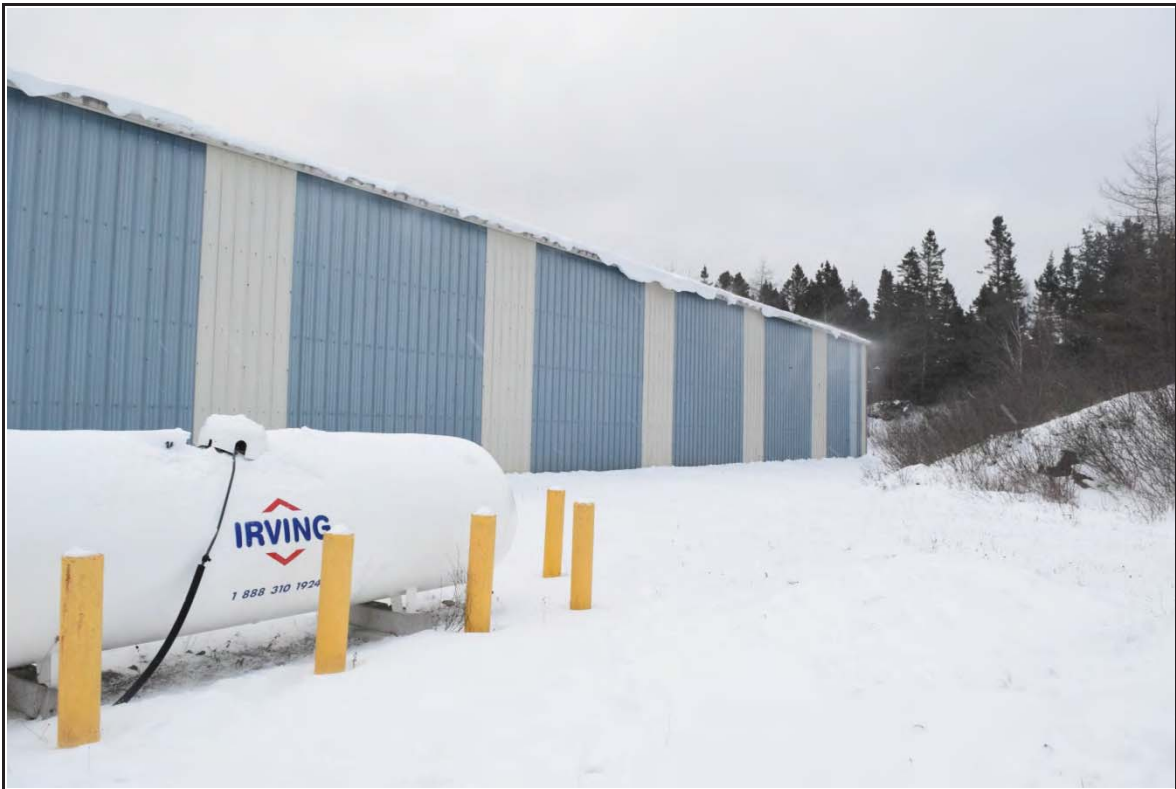
Photo 4: Partial South Elevation
