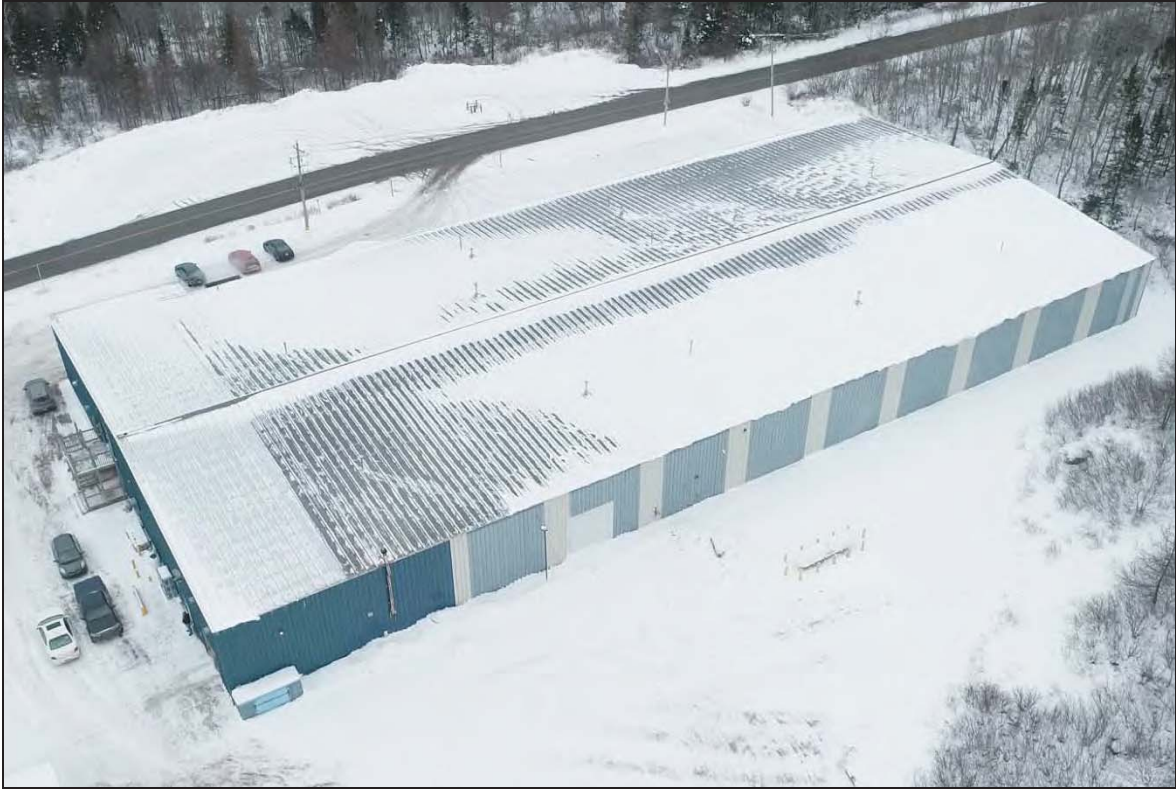
Photo 7: Building Roof and Surrounding Area
