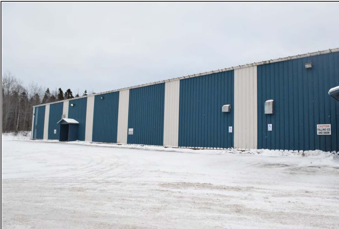
Photo 2: Partial North Elevation
