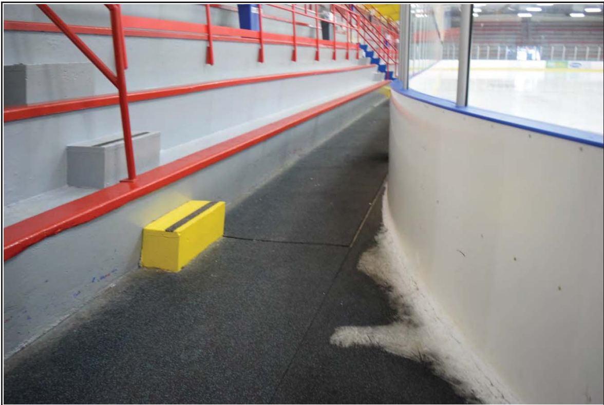
Photo 14: Typical Bleacher and Rink Area Finishes
