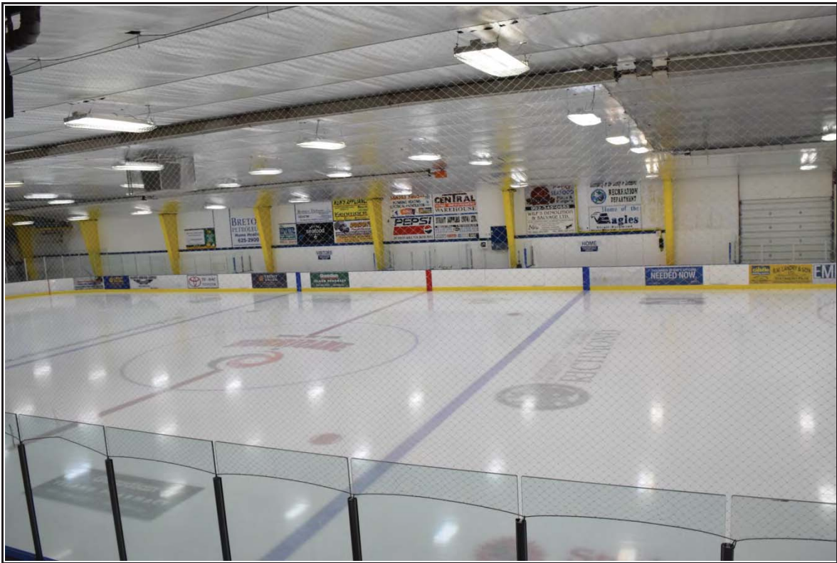
Photo 12: Arena Area, Dasher Boards, Lighting, Protective Nets, and Low-E Ceiling
