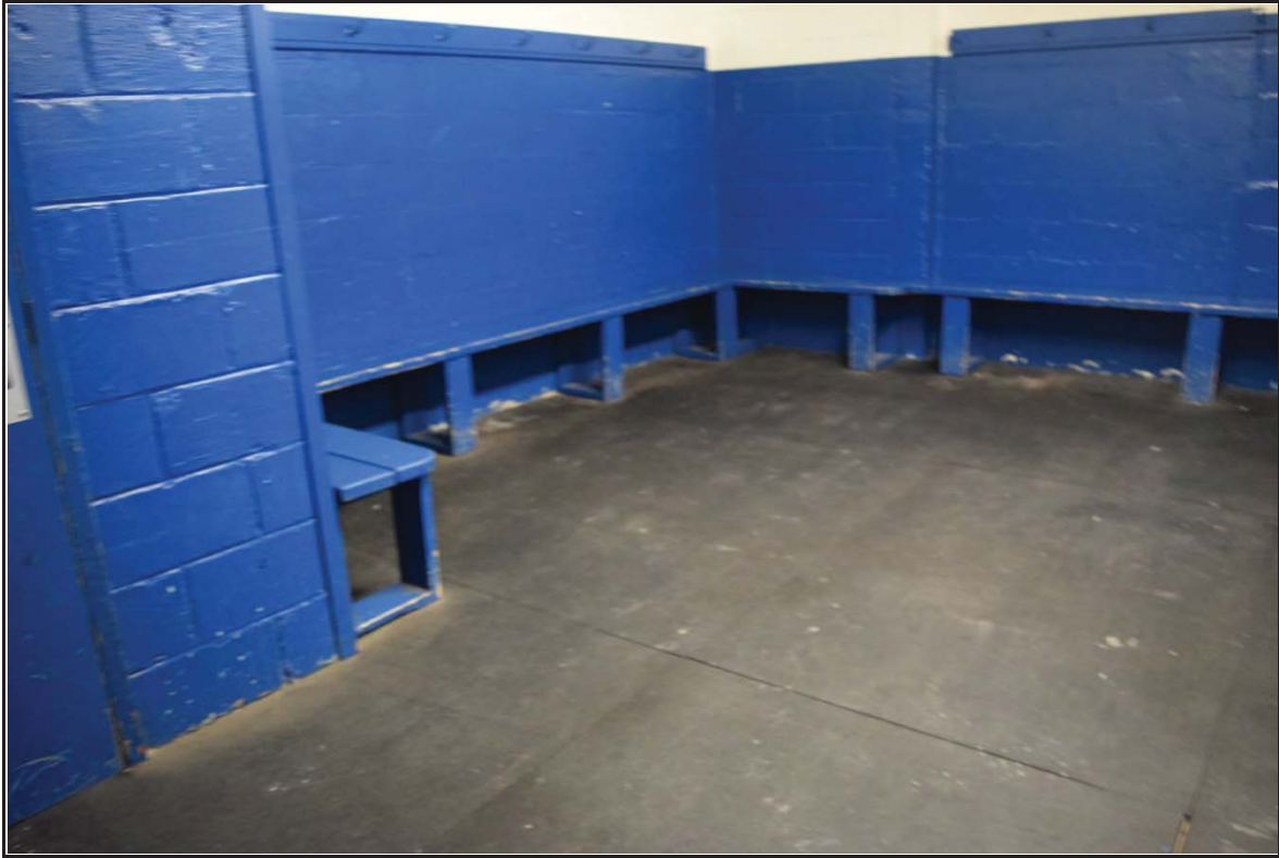
Photo 15: Changing Room #1 Finishes
