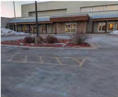
HE 14 | Accessible parking near front entrance
