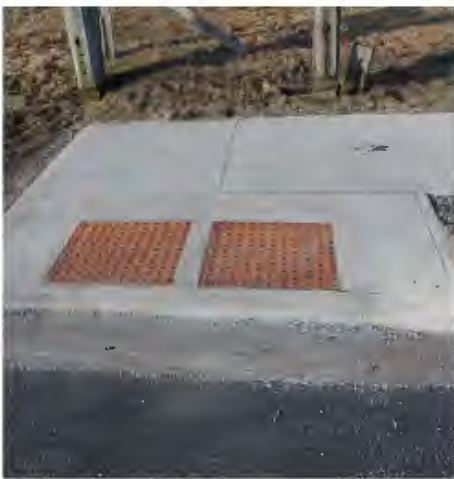
MS 3 | New TWSI at end of Arichat sidewalk
