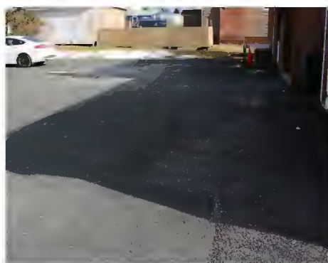
MB 18 | Accessible Parking - Back of Building
