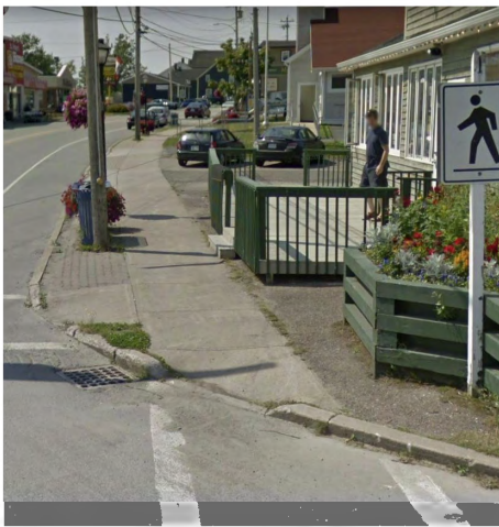
MS 8 | Dual curb cuts at crosswalk intersection
