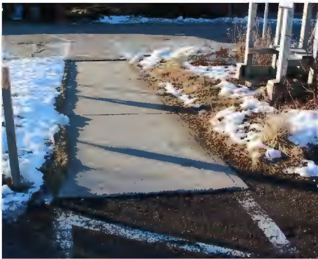
HE 6 | Walkway Leading from Parking to Front Entrance
