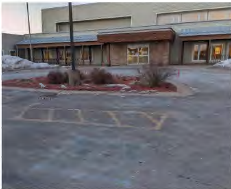
HE 14 | Accessible parking near front entrance
