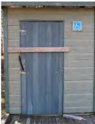
PA 4 | Accessible Washroom
