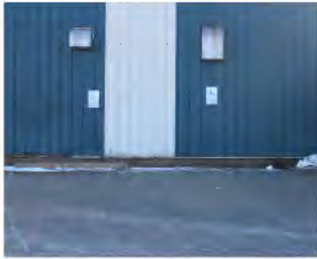
AR 1 | Accessible Parking Spaces Adjacent to Entrance
