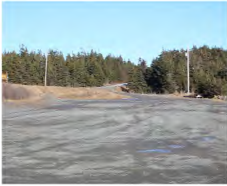
PA 5 | Parking Lot
