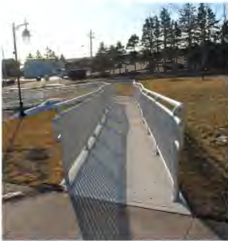
MB 5 | Ramp with TWSI along with upper and cane detectable lower rails
