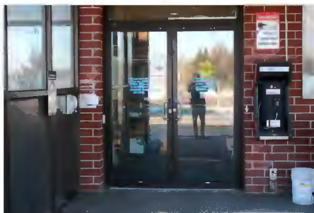
HE 7 | Main Entrance Door
