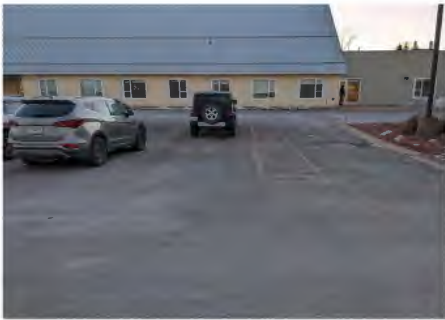
HE 13 | Access isle adjacent to accessible parking lot at Richmond Villa
