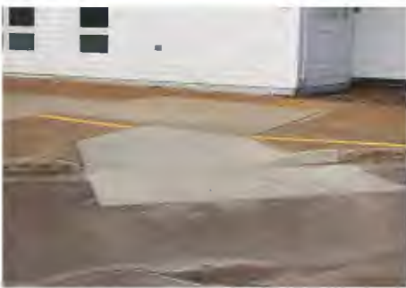
HE 9 | Curb Ramp from Parking to Walkway
