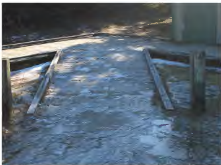
PA 7 | Sloped Walkway to Washroom and Change room Buildings
