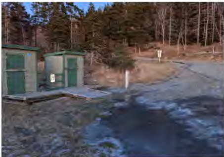
PA 10 | Outdoor accessible washrooms
