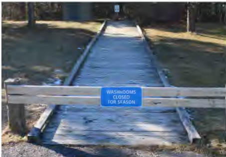
PA 3 | Ramp to Washrooms
