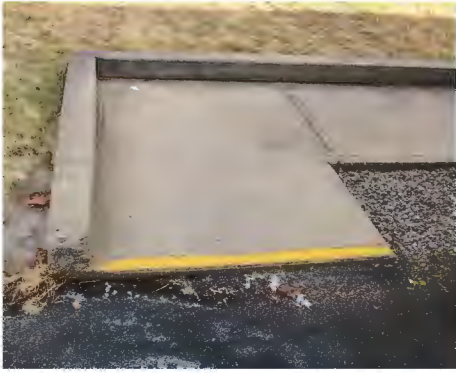
MB 19 | Accessible Walkway Threshold from Parking Lot
