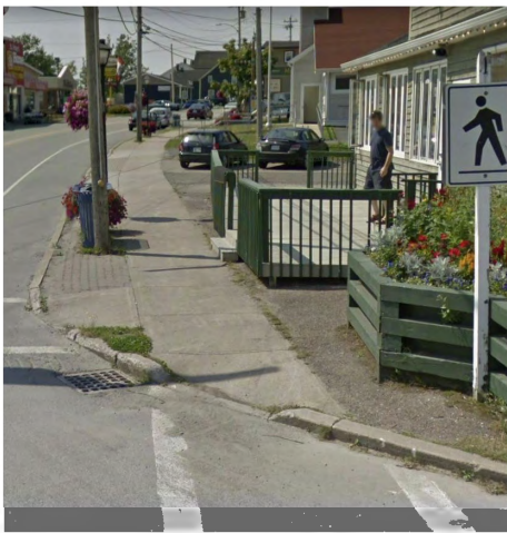
MS 8 | Dual curb cuts at crosswalk intersection
