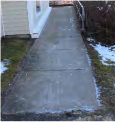
MB 11 | Accessible Ramp
