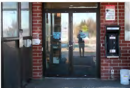
HE 7 | Main Entrance Door
