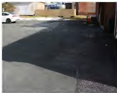
MB 18 | Accessible Parking - Back of Building
