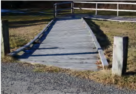
PA 2 | Sloped Walkway to Seating Area
