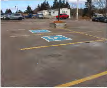
HE 8 | Accessible Stalls in Parking Lot
