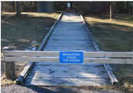
PA 3 | Ramp to Washrooms
