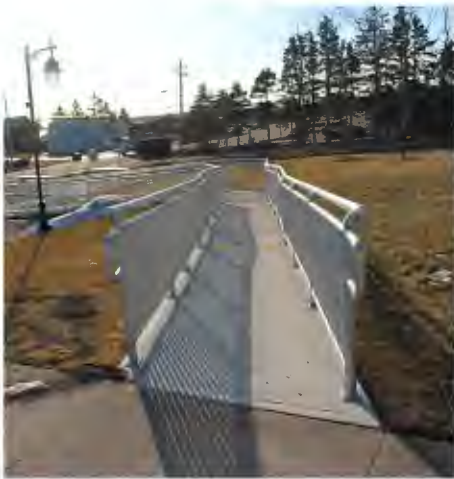
MB 5 | Ramp with TWSI along with upper and cane detectable lower rails
