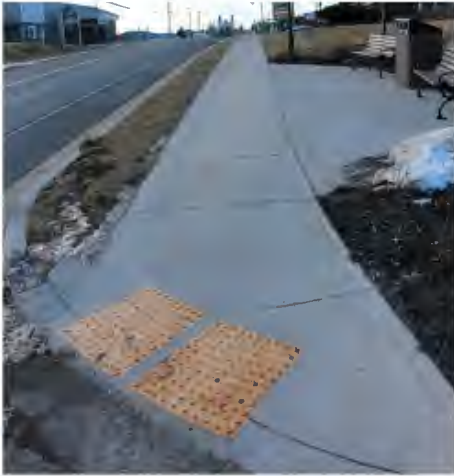
MS 1 | TWSI at end of sidewalk along with a rest area for pedestrians
