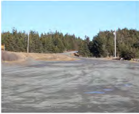
PA 5 | Parking Lot
