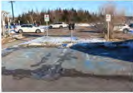
HE 4 | Accessible Parking Front of Building- Metered
