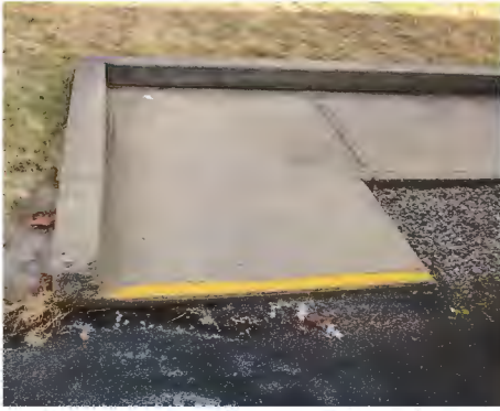
MB 19 | Accessible Walkway Threshold from Parking Lot
