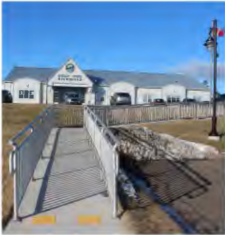
MB 4 | Path to Arichat main street from the Administration Building
