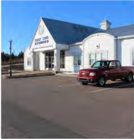
MB 1 | Richmond County Administration Building Upper Parking Lot
