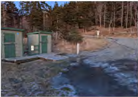
PA 10 | Outdoor accessible washrooms
