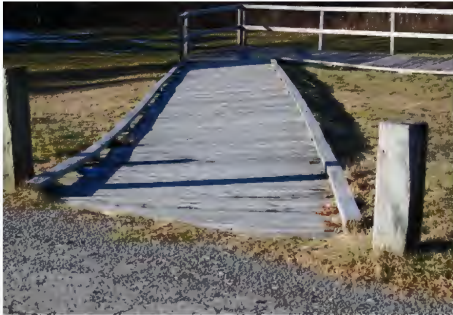
PA 2 | Sloped Walkway to Seating Area
