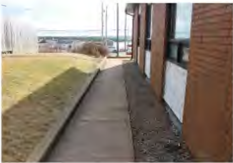
MB 20 | Walkway Leading to Front Entrance from Accessible Parking
