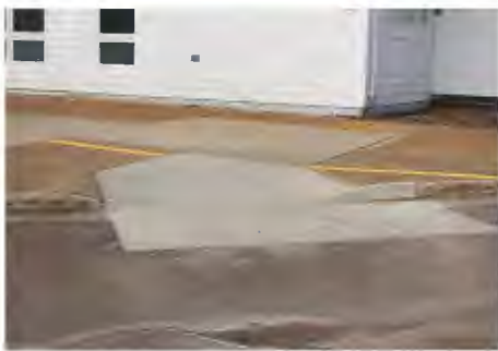
HE 9 | Curb Ramp from Parking to Walkway
