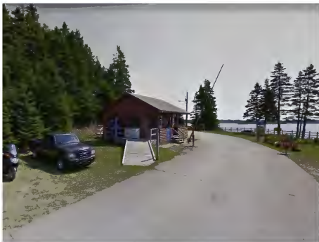
PA 12 | Access ramp at the Battery Park campground office
