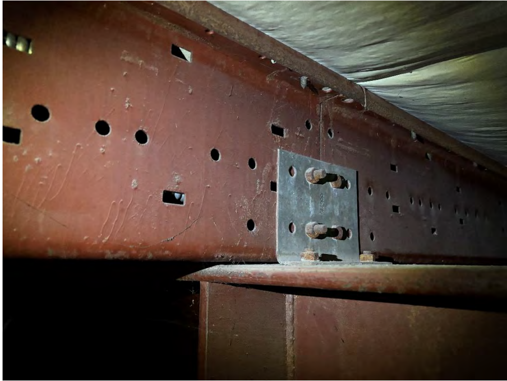
Photo 5 – Unpainted Roof Purlins in Storage Area on North Side of Arena in Excellent Condition.
