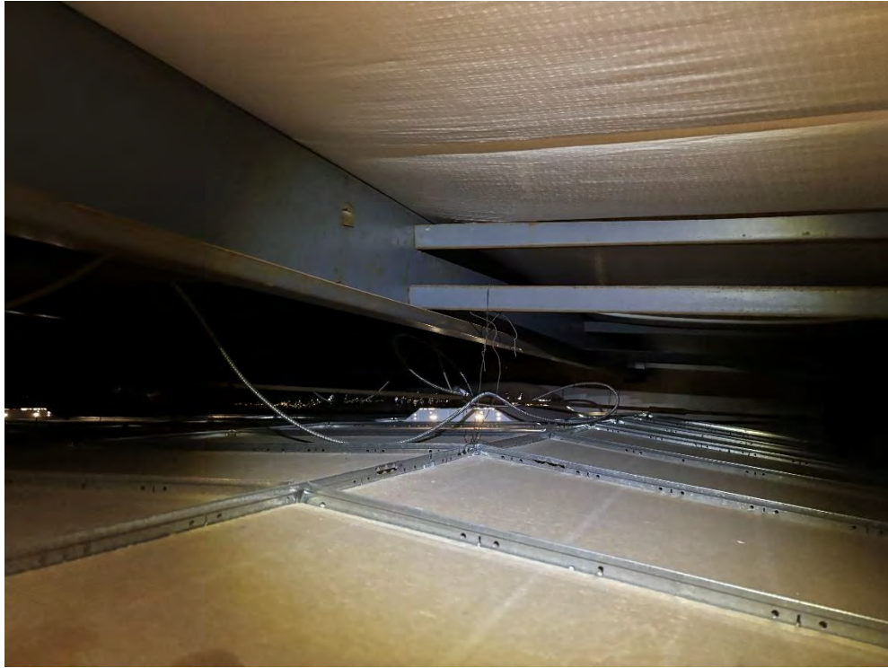
Photo 17 – Typical Roof Purlin in 1998 Addition with Two Rows of Purlin Bracing at Quarter Spans.
