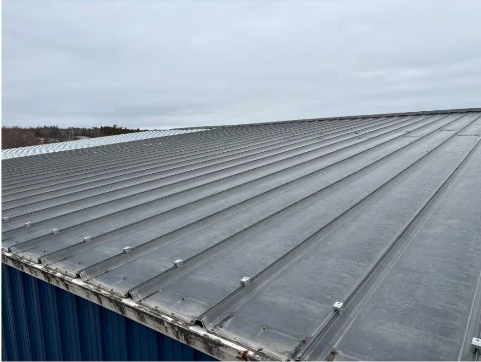
Photo 3 – View of Standing Seam Roof Panels from South Side of Building.
