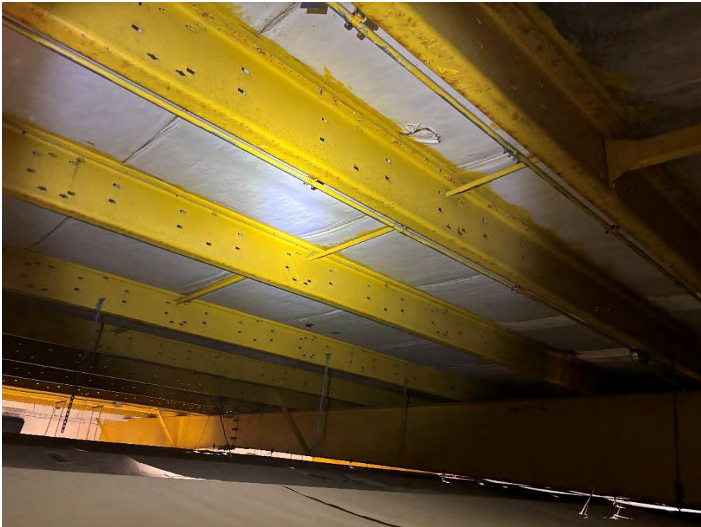
Photo 2 – Typical Roof Purlins with Top Flange Bracing at Midspan.
