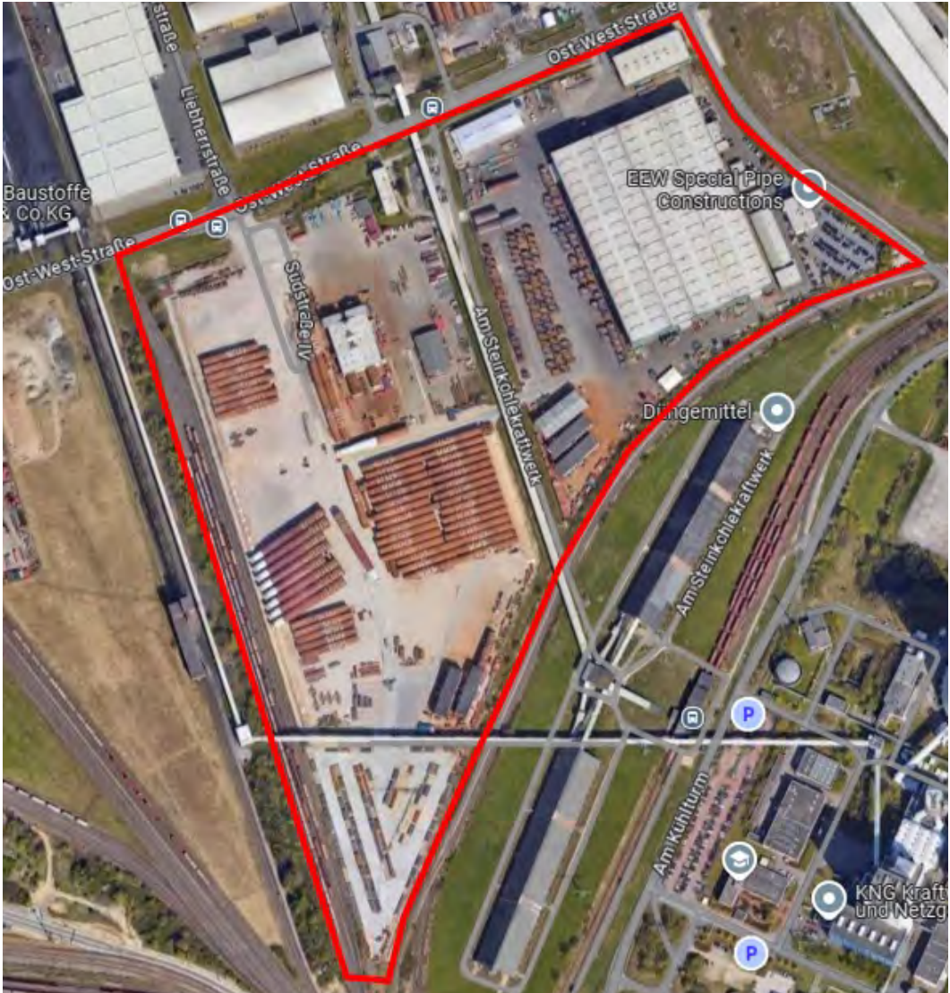
FIGURE 18: EEW MONOPILE MANUFACTURING - PORT OF ROSTOCK, GERMANY
