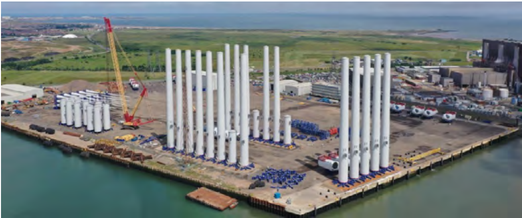
FIGURE 6: FIXED BOTTOM PORT, SOURCE: ABLE, UK
