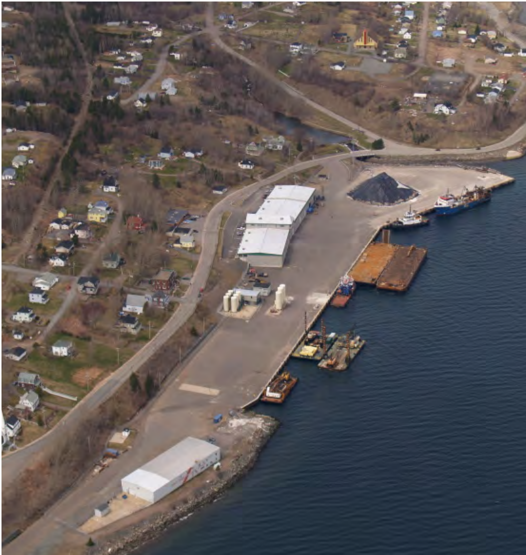
FIGURE 2: MULGRAVE MARINE TERMINAL, SOURCE STRAIT SUPERPORT CORPORATION
