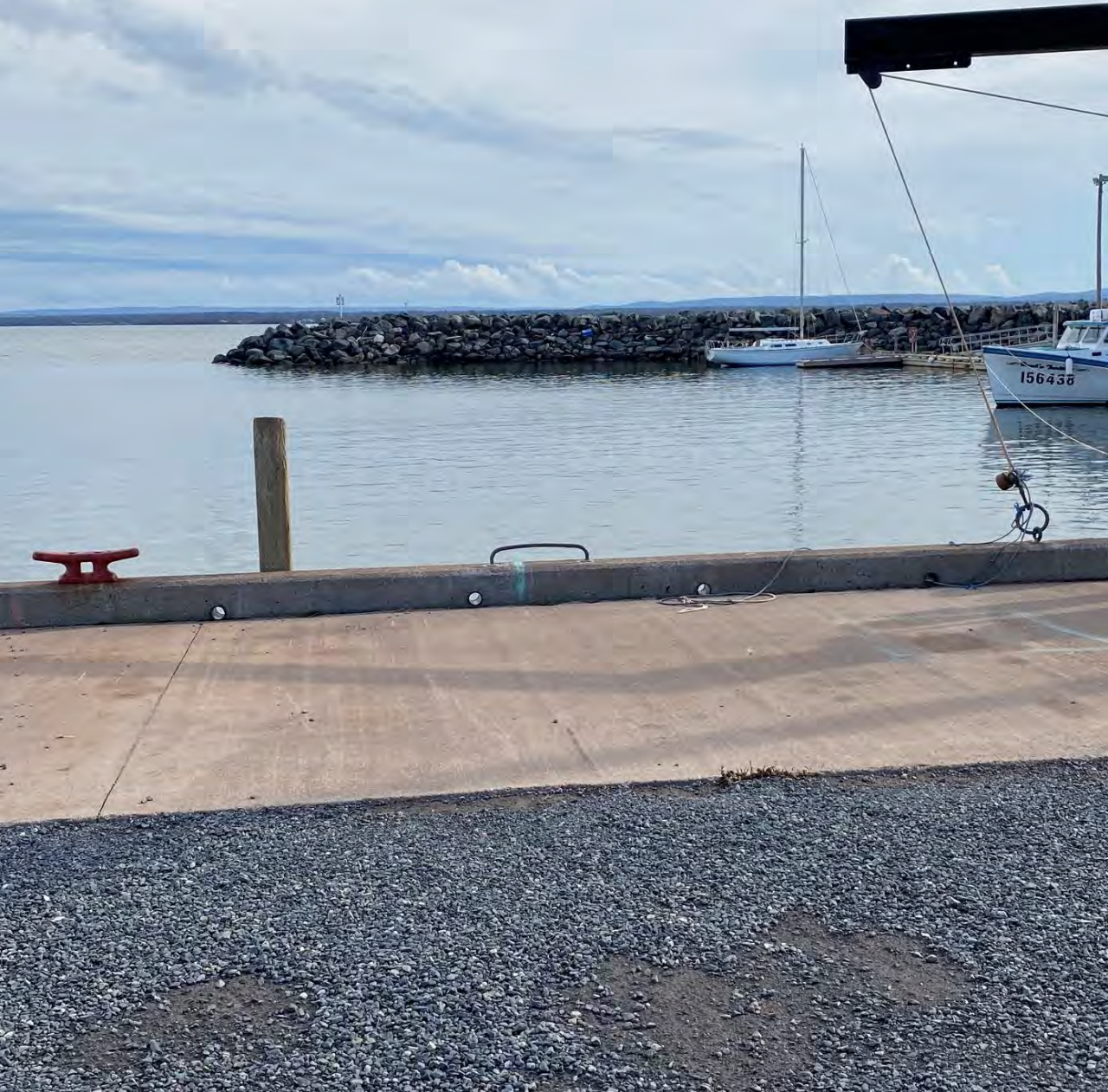
Cape John Wharf Normal Water Level
